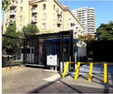
Image 8. US Embassy in Baku - rising wedge type road barrier in front of the entrance gate to the facility.
