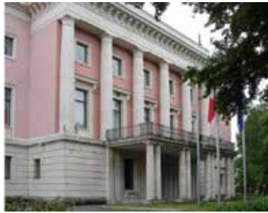
Image 14. Front facade of the Embassy of the Italian Republic in Berlin.
