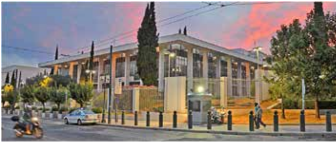
Image 12. US Embassy in Athens - zonal security in the form of static road barriers, high fencing, a permanent guard booth for law enforcement and road patrol.
