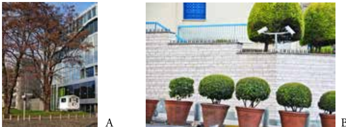
Image 3. Static posts as part of zonal protection in front of the Embassy of the Kingdom of the Netherlands in Berlin (A), freestanding protection posts and pots as part of passive zonal protection in front of the Israeli Embassy in Athens (B).
