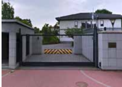
Image 9. Road barrier with rotating panel in the entrance area in front of the entrance to the Embassy and Residence of Japan in Warsaw.
