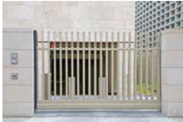
Image 11. Embassy of the Republic of Turkey in Berlin - openwork entrance gate in front of the garage exit, with movable security posts behind it (in the background).
