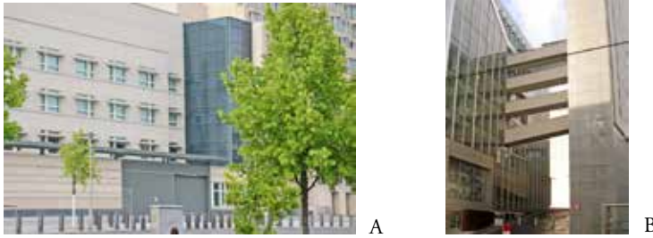
Image 7. Free-standing drop-down posts - in front of the entrance gate to the car park of the US Embassy in Berlin (A), within the entrance to the inner courtyard of the Embassy of the Kingdom of the Netherlands in Berlin (B).
