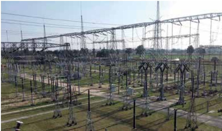
Fig. 2. 400/110 kV high-voltage switching station.
