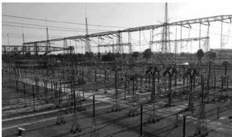
Fig. 2. 400/110 kV high-voltage switching station.
